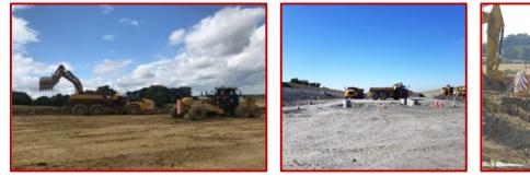
In this way, earthmoving continued at an efficient pace with two 50t excavator teams whilst ensuring the integrity of the monitoring points.
