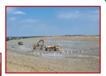
Excavated material was hauled along a purpose-built haul road to the deposition site in a meander of the Oxford Canal, where the material was stored in 10m high stockpiles for reuse in the HS2 main works.
